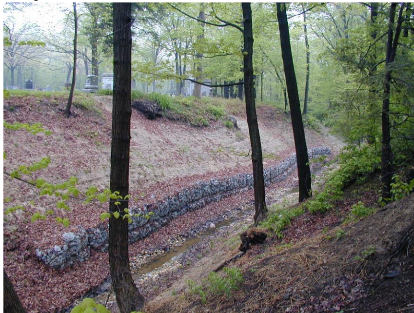
A restored Ravine: Improved light penetration, decelerated water in the channel, slope planted with native species plants, e
