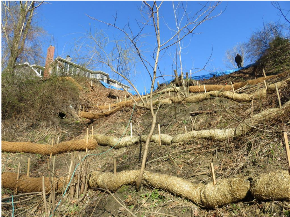
Contour wattling on a steep hillside.
